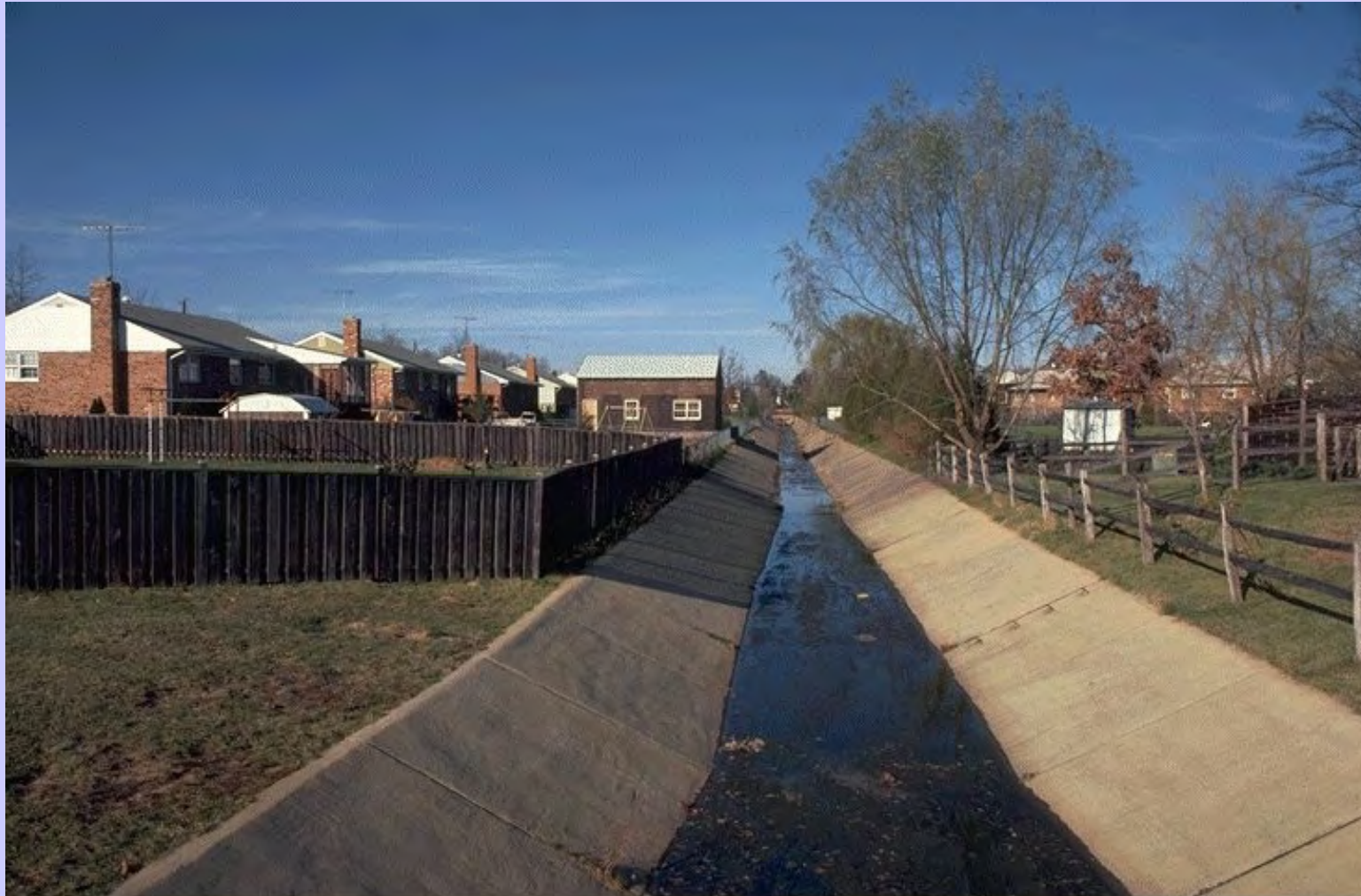
Fig. 3.10 – Stream channelization. Instream modifications, such as uniform cross section and armoring, result in ecological decline.
